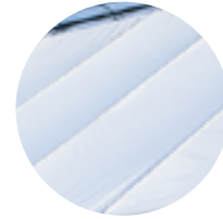
Roof membrane (AR 420).
