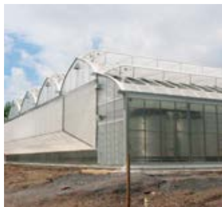
Mechanical ventilation (cooling pad)
