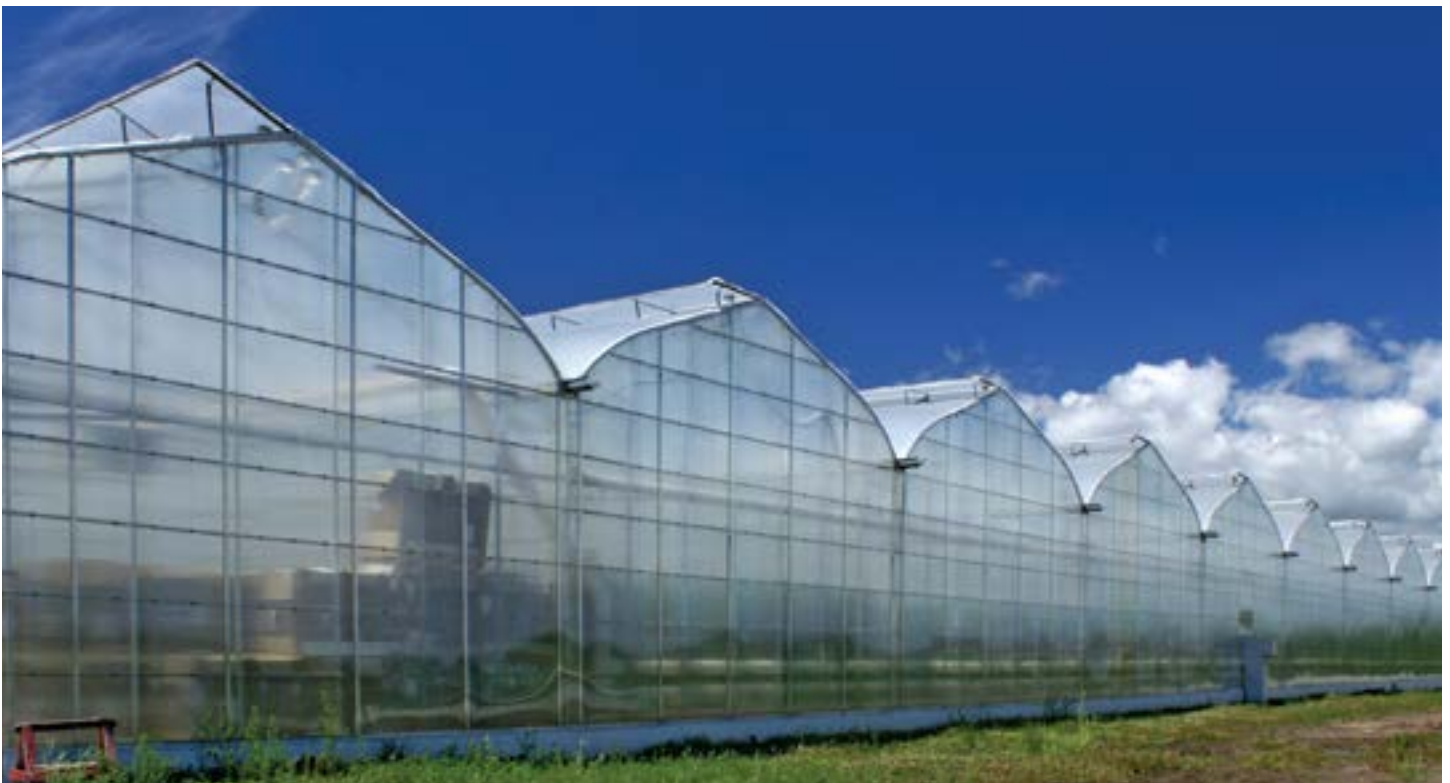
8 mm, double wall polycarbonate panels: this rigid covering offers excellent durability and good insulation.
