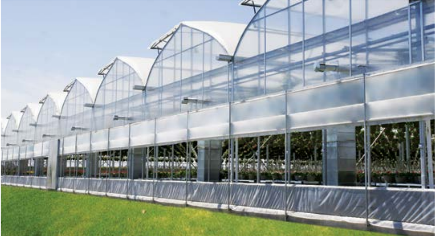
Double polyethylene films 7.2 mil: this option includes the blower and connections.
